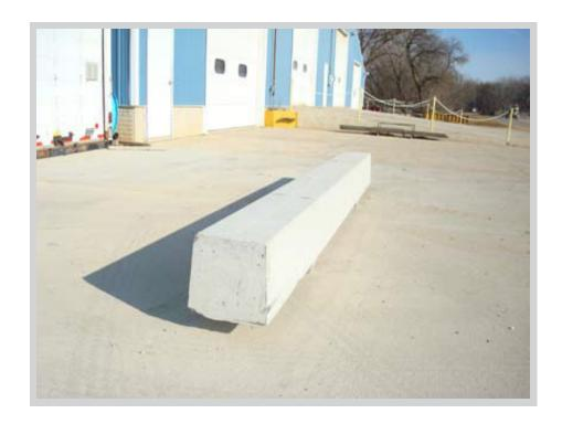
This is our standard beam. The common use is for supporting hog & cattle slats. It is designed to set in wall pockets (min. depth of 4") and on columns (min. surface 6").
